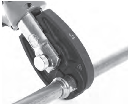
Figure 9 – Placing Jaws Around Fitting
